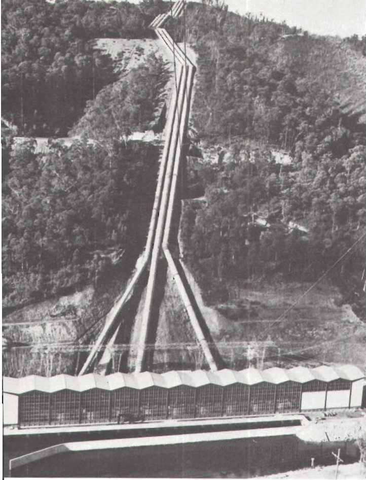
A view of the Murray 1 power station. Waters of the Snowy River are captured at Island Bend and diverted to the power station via the Geehi Reservoir.
