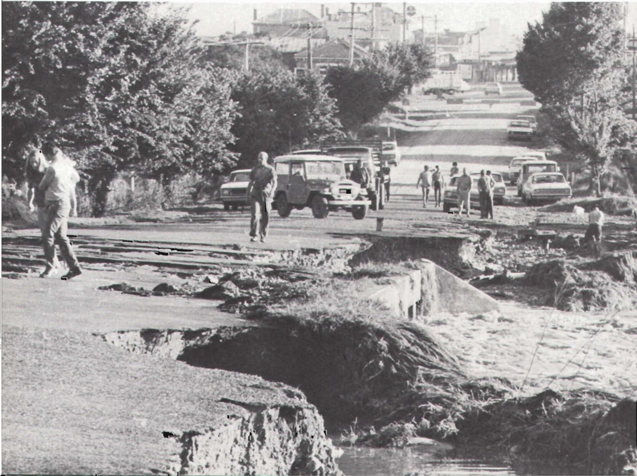
An example of the damage caused by flooding in East Gippsland during February 1971. This is a washed out section of the Princes Highway at Orbost. The Herald and Weekly Times Ltd
